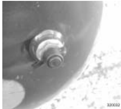
Test connection on the compressed air tank for brakes
